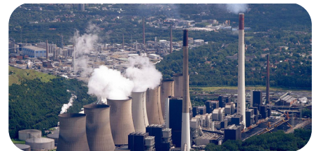
A thermal power station
